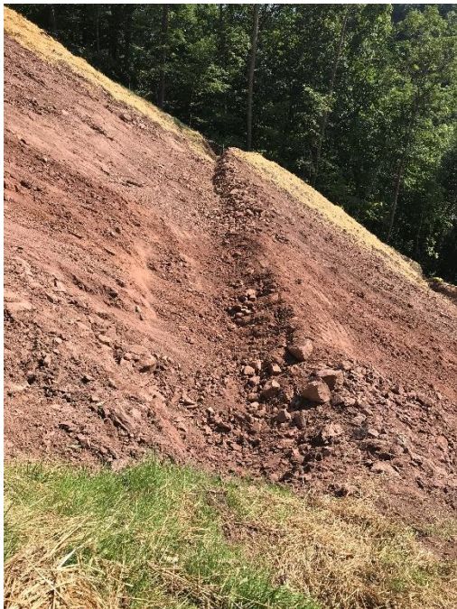
Fig. 3 Area near station # 12029+94
