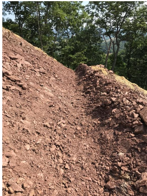
Fig. 4 Area near station # Area near station # 12028+97
