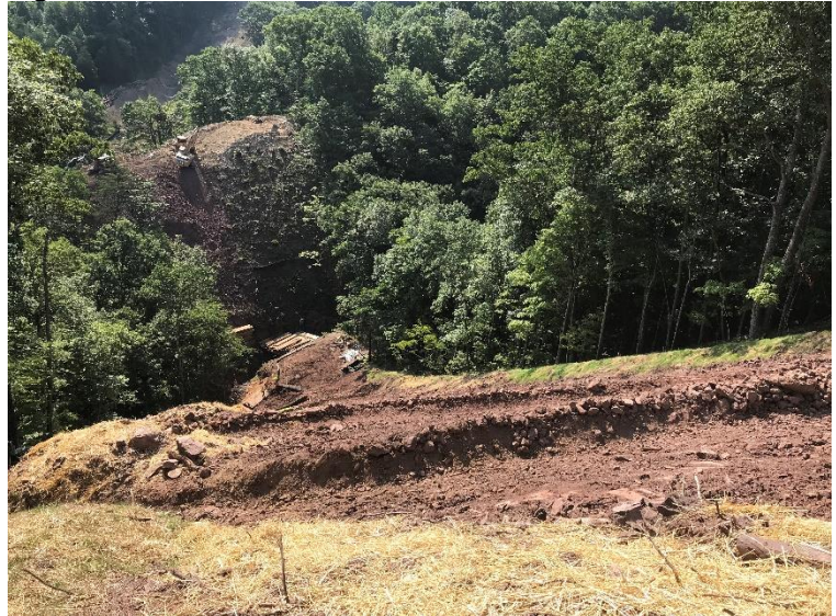
Fig. 2 Area above stream 40
