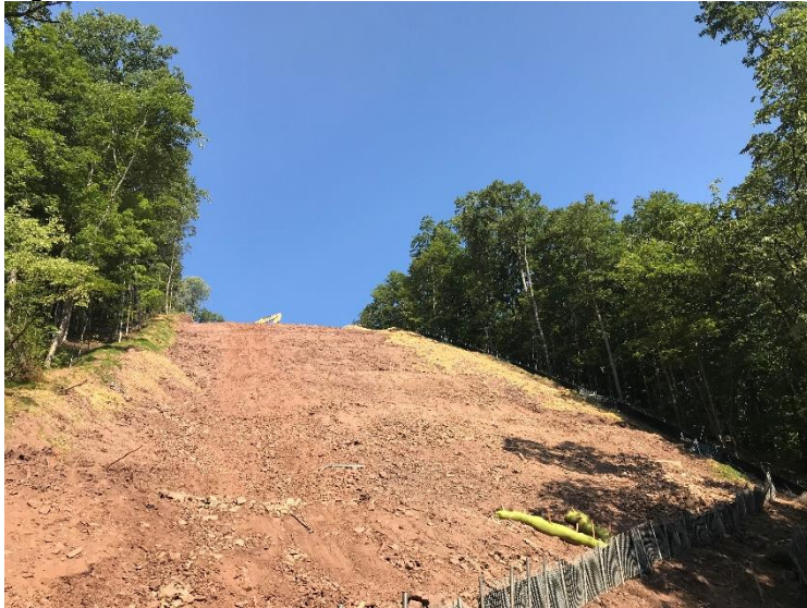
Fig. 1 Area near Mile Post 227.9
