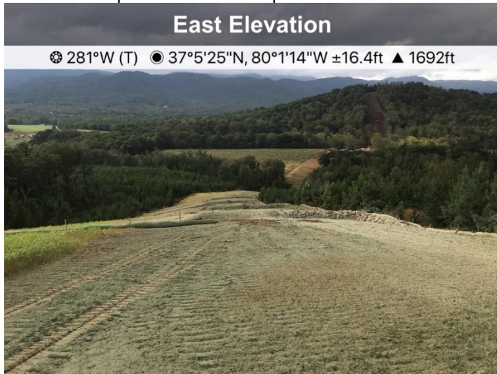
Fig. 3 At St# 13431 permanent bars in place and stabilized.
