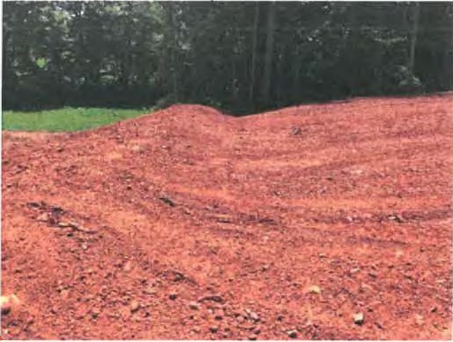
Fig. 5 Waterbar, typical (Area 2)
