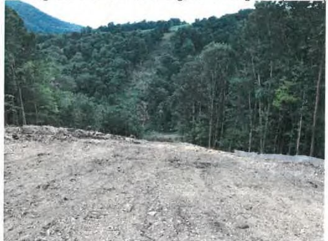
Fig. 8 Looking down to Rt 42 crossing, ahead of grade (Area 3)
