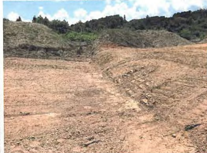
Fig. 4 Water Bar installation (Area 2)
