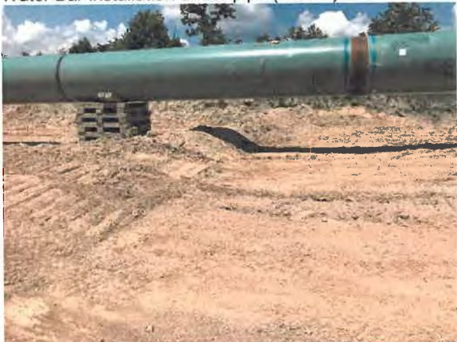
Fig. 3 Water Bar installation under pipe (Area 2)
