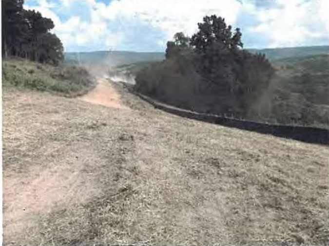
Fig. 3 Area above Mountain Lake Rd, ahead of grade (Area 3)
