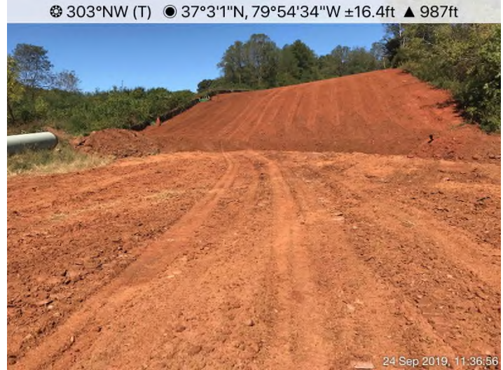
Fig. 8: STA 13908+00 – Final grading in progress. Spreading topsoil and re-establishing grade to existing contours.
