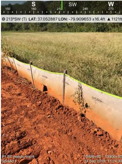
Fig. 7: STA 13906+55 – SSF maintenance need.
