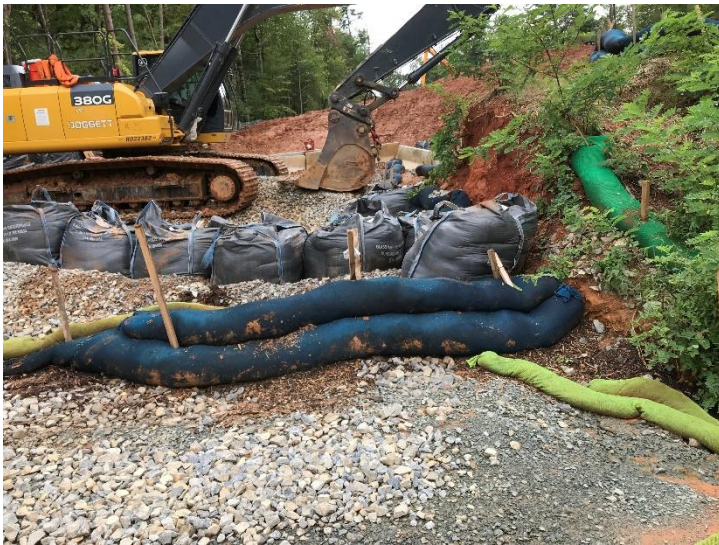
Fig. 3 MP255.40 Cahas Mtn Rd, additional controls have been installed at CE.
