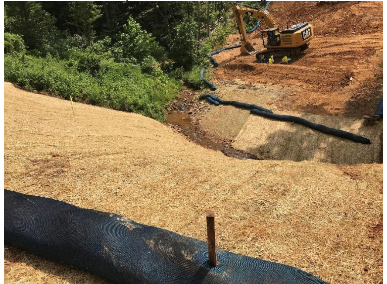
Fig. 4 Observed matted slope installed above designated stream S-IJ 4
