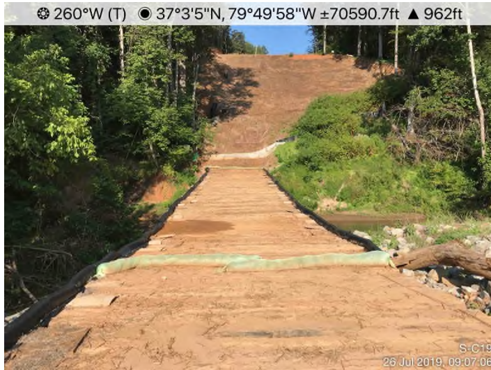
Fig. 3: Stream S-A40 – Controls in place and functioning properly.
