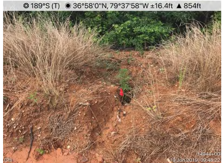
Fig. 4: STA 14944+00 – CFS maintenance needed. Repair and stabilize diversion berm.
