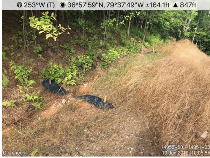
Fig. 7: STA 14951+00 to 14953+50 – CFS maintenance needed.
