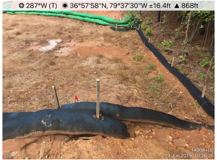
Fig. 8: STA 14967+00 – CFS maintenance needed.
