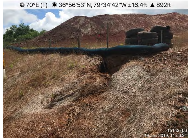
Fig. 12: STA 15143+00 – CFS maintenance needed.
