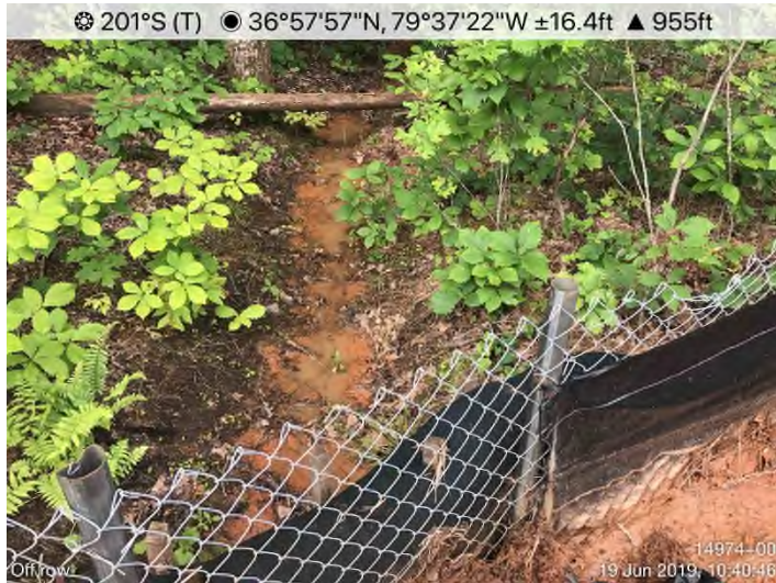
Fig. 11: STA 15126+00 – CFS/P1 maintenance needed.
