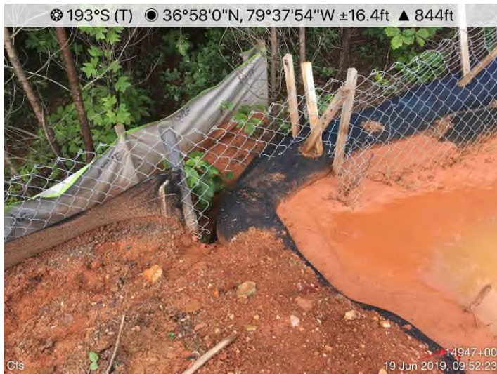
Fig. 7: STA 14951+00 to 14953+50 – CFS maintenance needed.
