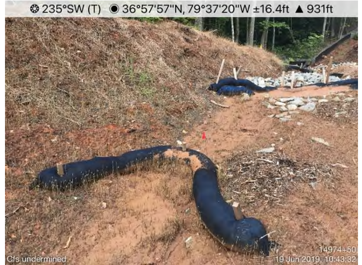
Fig. 12: STA 15143+00 – CFS maintenance needed.
