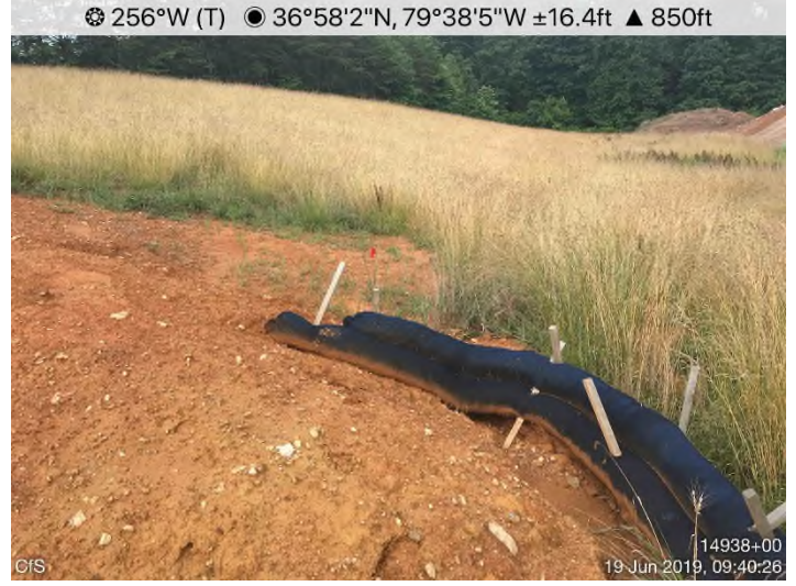
Fig. 4: STA 14944+00 – CFS maintenance needed. Repair and stabilize diversion berm.
