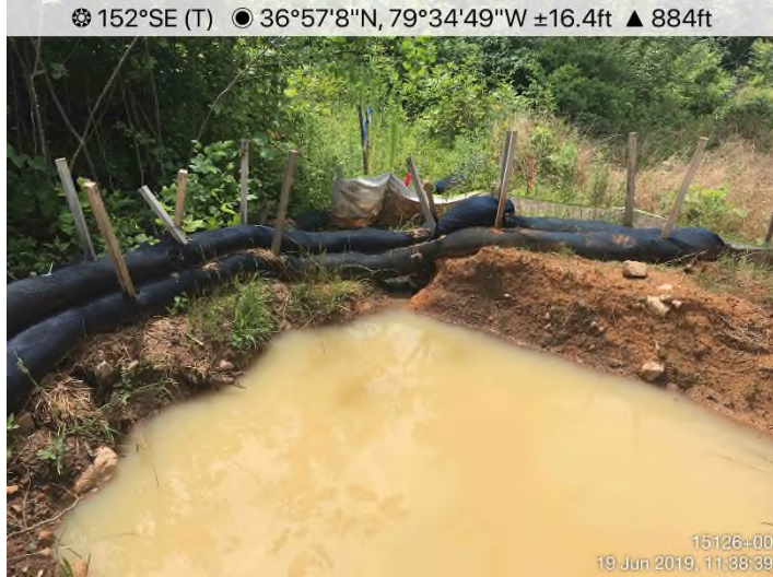
Fig. 11: STA 15126+00 – CFS/P1 maintenance needed.
