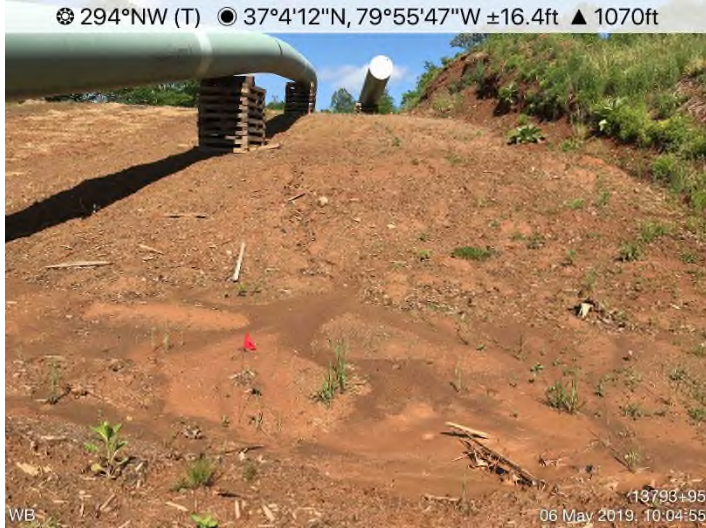
Fig. 3: STA 13793+95 – Stabilize area upslope of waterbar.
