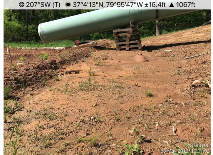
Fig. 4: STA 13793+95 – Waterbar does not extend to perimeter controls/flow diverting around waterbar.
