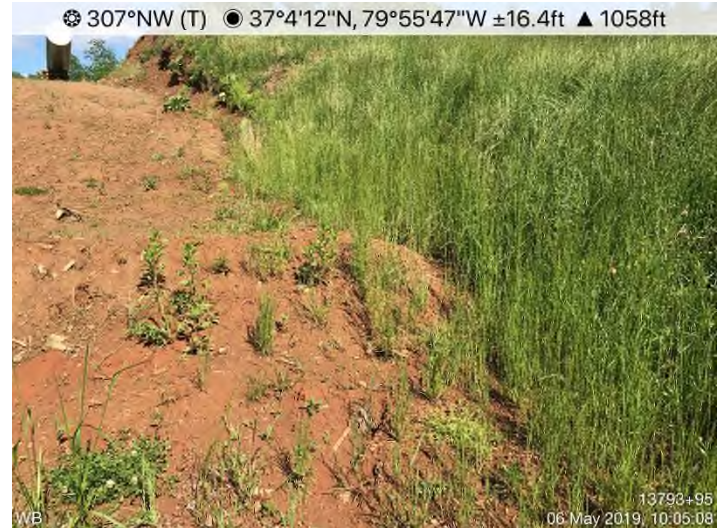
Fig. 4: STA 13793+95 – Waterbar does not extend to perimeter controls/flow diverting around waterbar.
