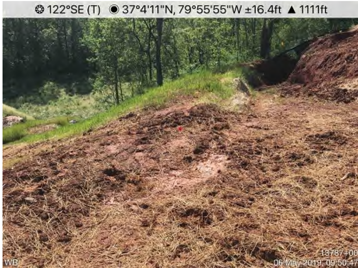
Fig. 3: STA 13793+95 – Stabilize area upslope of waterbar.
