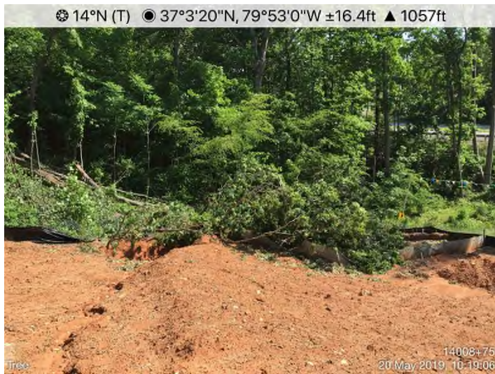
Fig. 3: STA 14008+75 – Remove fallen tree. Repair ECDs.
