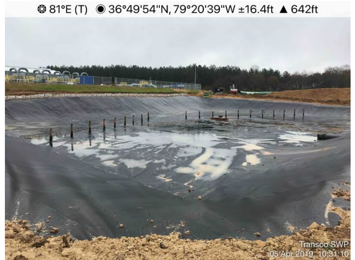
Fig. 4: Transco Stormwater Pond – Liner and baffle installation.
