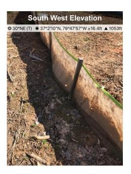
Fig. 3 St#14353+17 bank stabilization matting has fallen off slope
