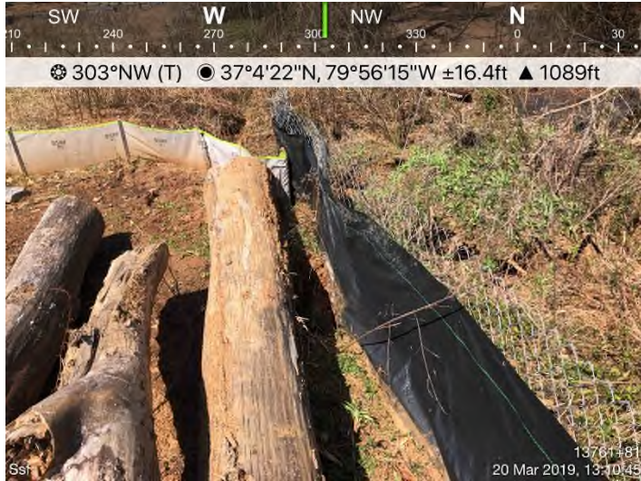
Fig. 3: STA 13761+87 – SSF undermined.
