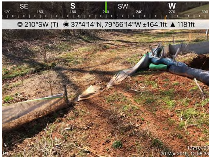
Fig. 3: STA 13761+87 – SSF undermined.
