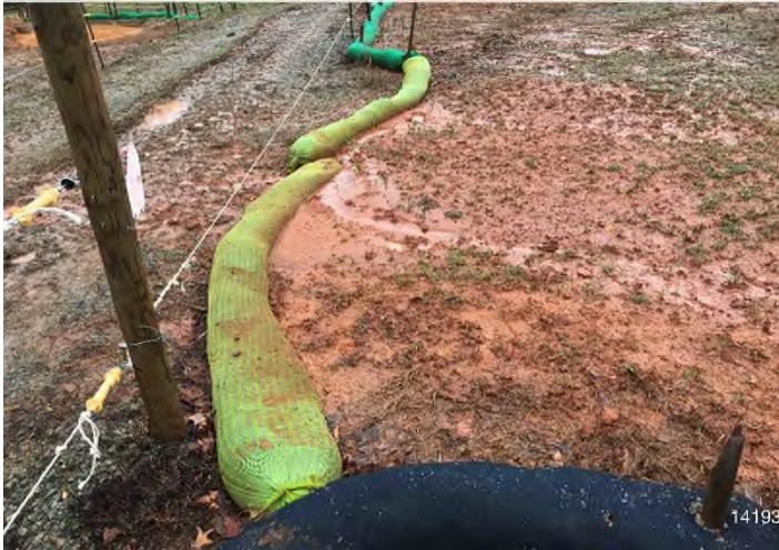
Figure 3: STA 14193+00 – CFS wattle in need of maintenance.
