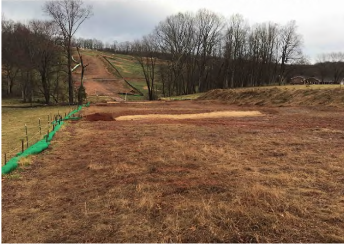
Figure 3: STA 14193+00 – CFS wattle in need of maintenance.
