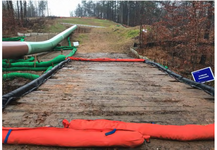
Fig. 4: Stream S-KL36 – Controls in place and properly functioning along Stream S-KL36 crossing.
