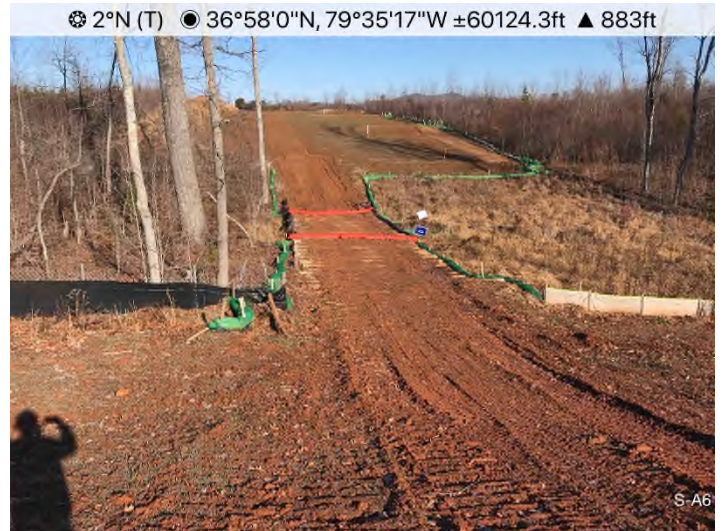
Fig. 4: STA 13867+57 – Controls in place and properly functioning. Area stabilized with vegetation.
