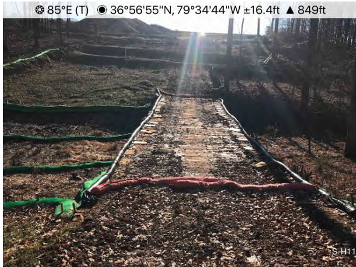
Fig. 3: STA 13860+00 – Controls in place and functioning above Stream S-C17. Area stabilized with vegetation.
