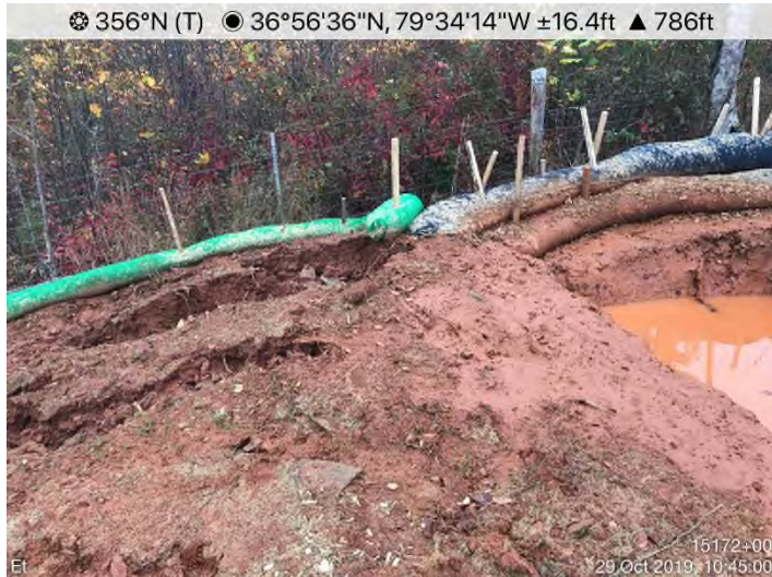
Fig. 3: STA 15169+58 – Sediment off ROW. Controls overtopped.
