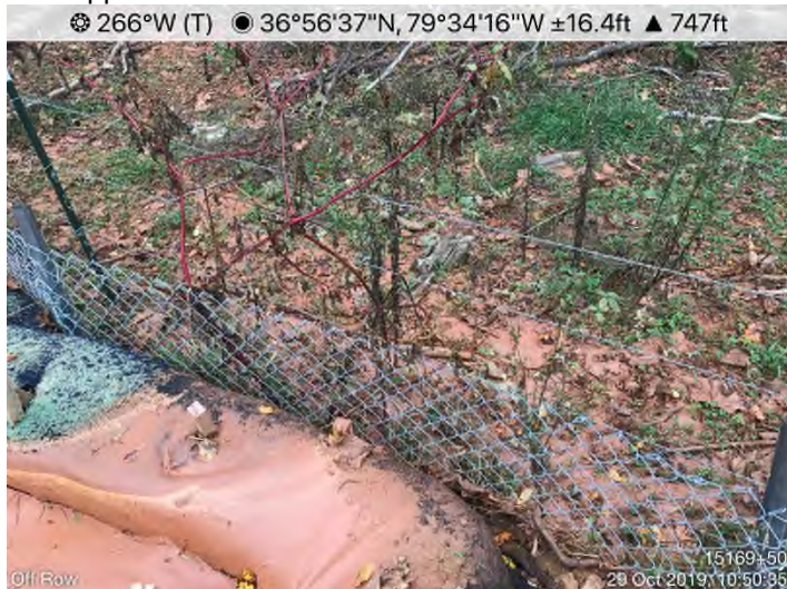
Fig. 3: STA 15169+58 – Sediment off ROW. Controls overtopped.
