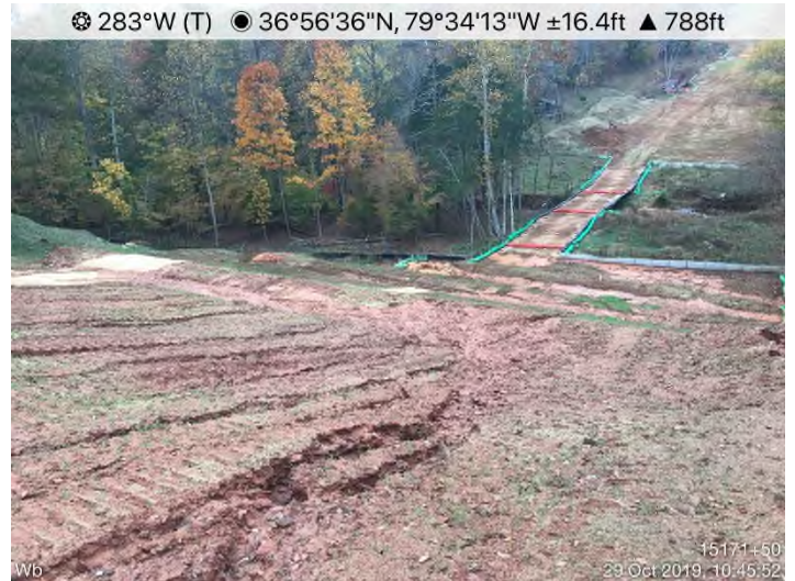
Fig. 4: STA 15169+58 – CFS overtopped. Maintenance needed.
