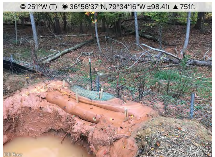
Fig. 4: STA 15169+58 – CFS overtopped. Maintenance needed.
