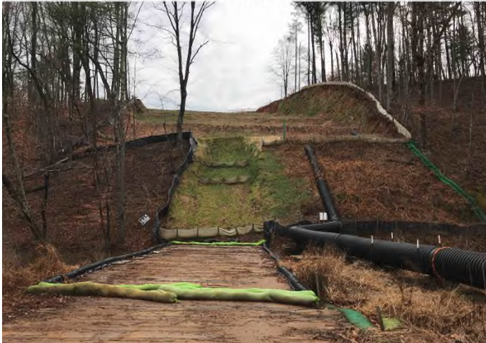
Fig. 3: Wetland W-CD5 – Controls in place around wetland crossing. Area stabilized.
