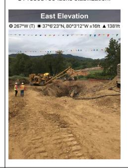
Fig. 3 Near MP 246.7 stabilization and permanent bars have been installed.
