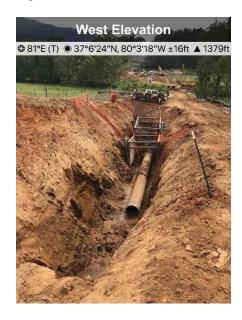
Fig. 2. Active bore site near GH-7, stockpile near ST13308+99 lacks stabilization.
