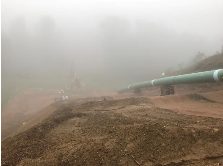
Fig. 3 In the area of MP246.43 St# 13012+00 area has been matted.
