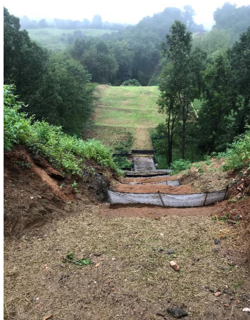
Fig. 4 MP 252.21 St#13317+00 – 13320+00 blanket matting has been installed.
