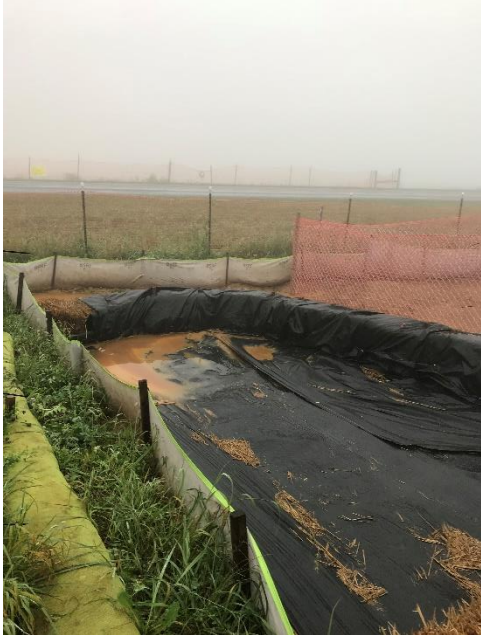
Fig. 1 MP 246.47 St#13014+00 dewatering structure in place
