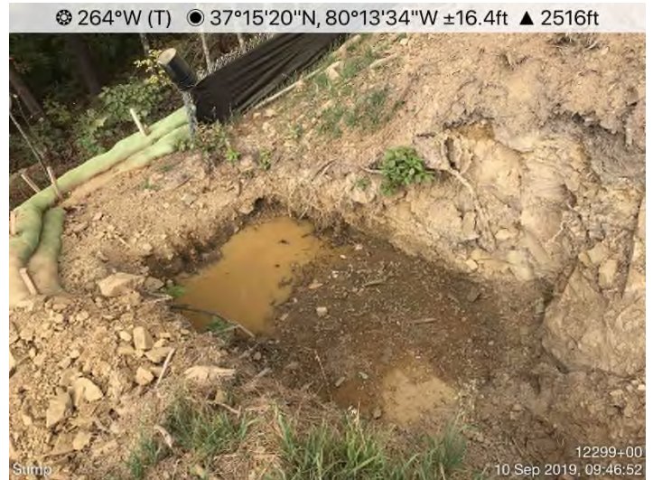
Fig. 4: STA 12361+10 – SSF undermined.
