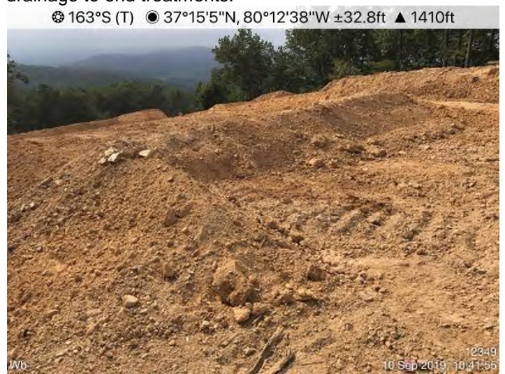
Fig. 8: STA 12321+00 to 12356+00 – Waterbars do not extend full length of ROW. Waterbars do not have positive drainage to end treatments.
