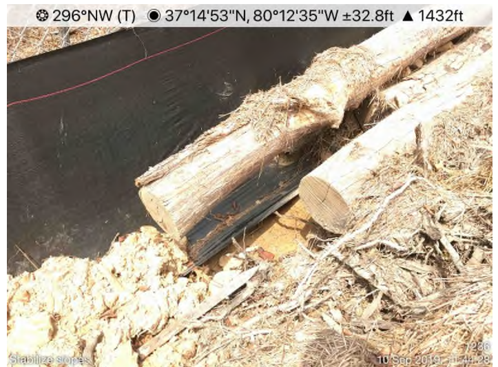
Fig. 4: STA 12361+10 – SSF undermined.
