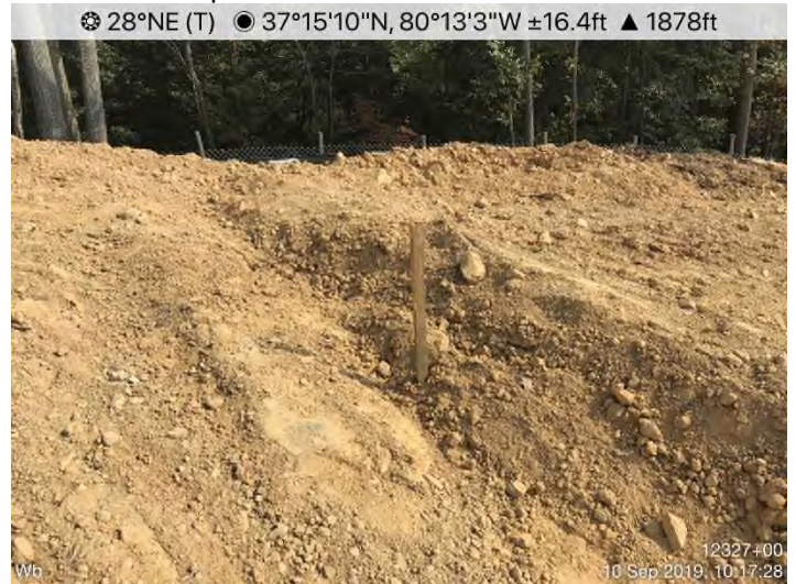
Fig. 8: STA 12321+00 to 12356+00 – Waterbars do not extend full length of ROW. Waterbars do not have positive drainage to end treatments.
