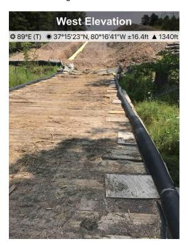
Fig. 2 At designated stream MM-13 ECD's are in place and functioning.
