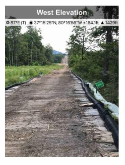
Fig. 3. At designated stream S-C29 ECD's are in place and functioning.
