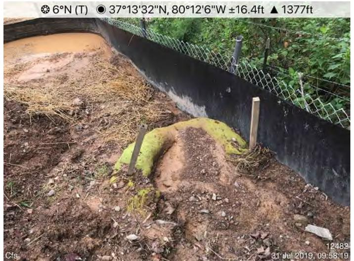
Fig. 7: **STA 12483+00** – Sump maintenance needed.
