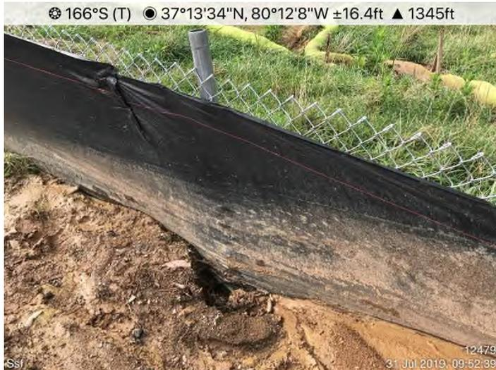
Fig. 2: **STA 12480+00** – SSF maintenance required.
