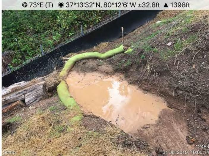
Fig. 8: **STA 12483+00** – Waterbar repair needed.
