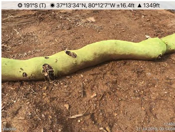
Fig. 4: **STA 12481+00** – Replace damaged bridge wattle.
