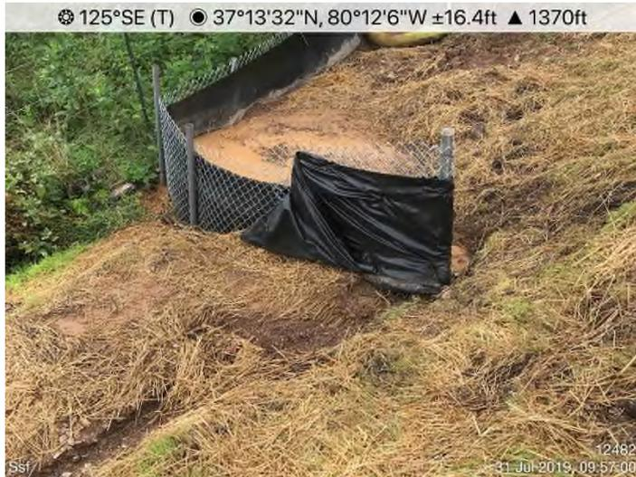
Fig. 6: **STA 12482+00** – CFS maintenance needed.
