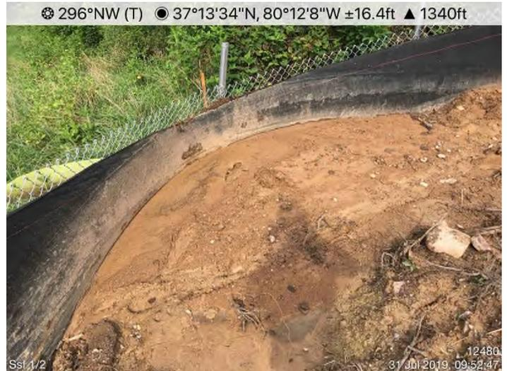
Fig. 3: **STA 12480+00** – Replace damaged bridge wattle.
