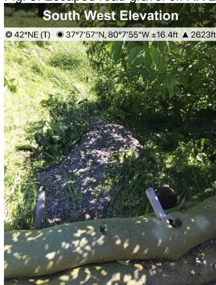
Fig. 3. Escaped road gravel off AR 288.
