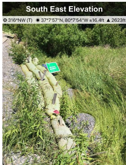
Fig. 1 Escaped road gravel off AR 288.
