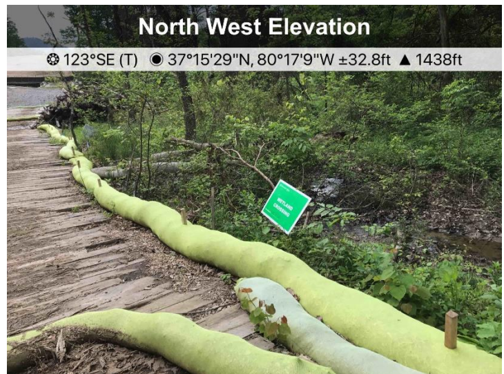
Fig. 4. At designated wetland W-F9-PFO, ECD's are in place.
