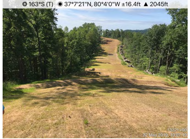
Fig. 4: STA 13245+00 – Controls in place. Area stabilized with erosion fabric/Earth Guard.
