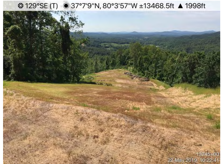
Fig. 4: STA 13245+00 – Controls in place. Area stabilized with erosion fabric/Earth Guard.
