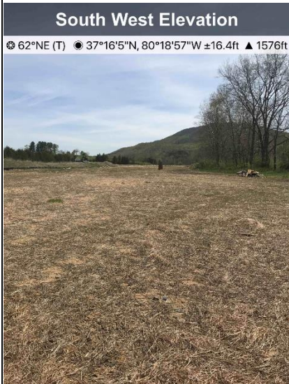
▪ Fig. 1 ATWS 473 temporarily stabilized
