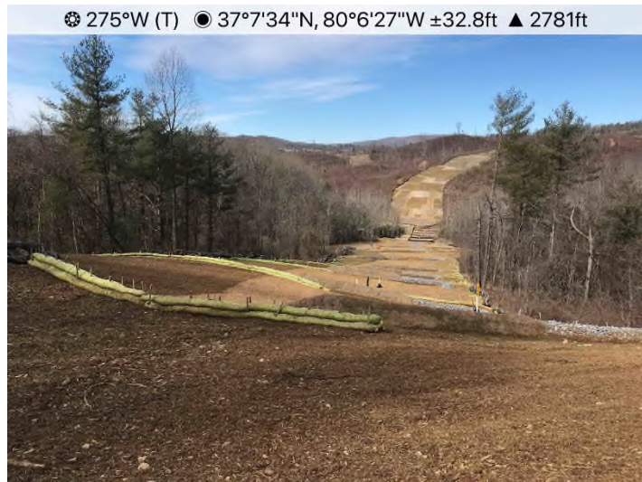
Figure 3: STA 13072+00 – Controls in place and functioning properly.
