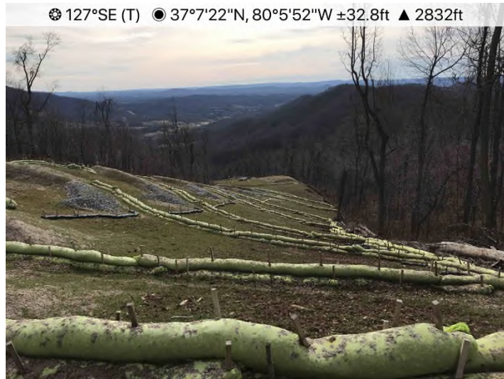
Figure 3: STA 13072+00 – Controls in place and functioning properly.
