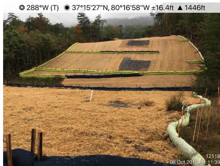
Fig. 3: STA 12117+62 – Controls in place. Area stabilized with straw and erosion matting.
