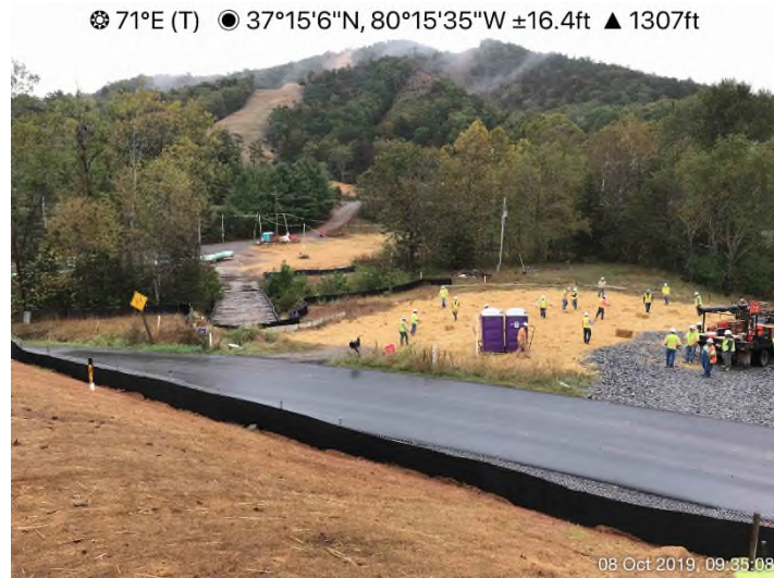
Fig. 3: STA 12117+62 – Controls in place. Area stabilized with straw and erosion matting.
