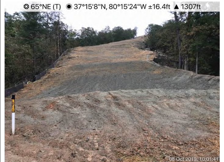
Fig. 4: Stream S-MM11 – Controls in place. Area stabilized with straw and erosion matting.
