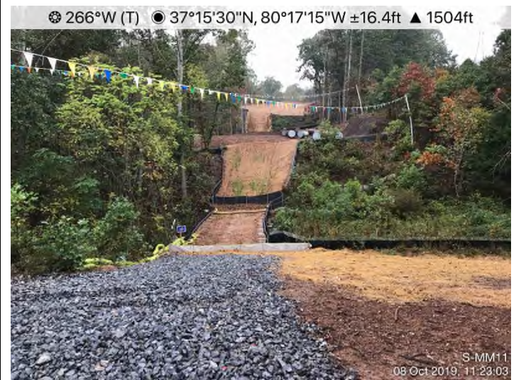
Fig. 4: Stream S-MM11 – Controls in place. Area stabilized with straw and erosion matting.
