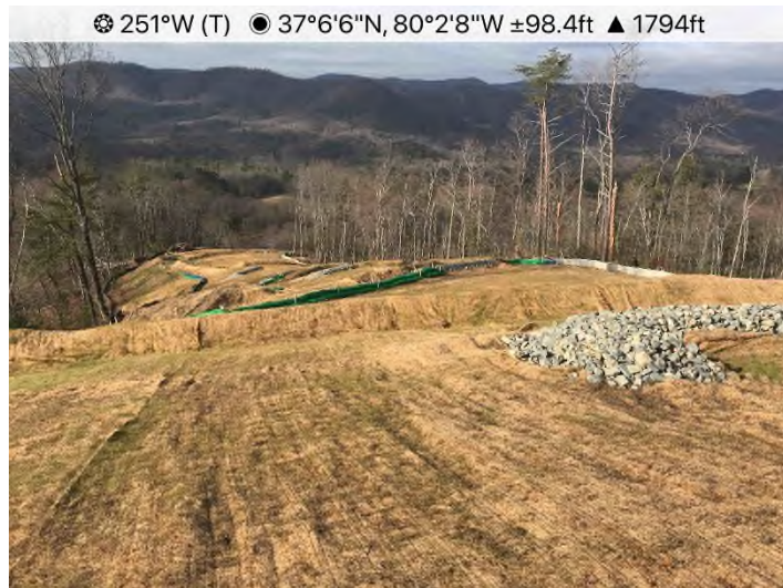
Figure 3: STA 13371+00 – Controls in place and functioning properly. Area stabilized with erosion matting.
