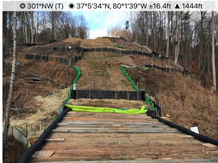
Figure 3: STA 13371+00 – Controls in place and functioning properly. Area stabilized with erosion matting.
