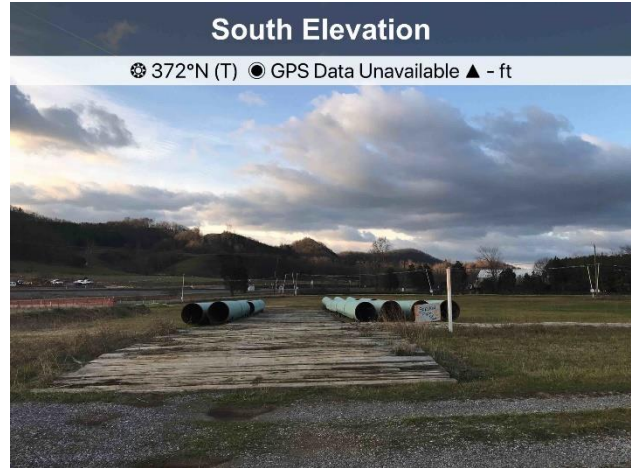
Fig. 2. At ATWS 645 and 645A, ECD's are in place.
