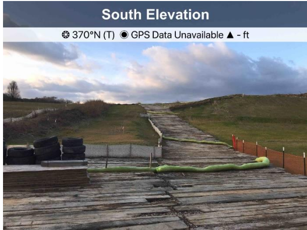
Fig. 1. At ATWS 645 and 645A, ECD's are in place.
