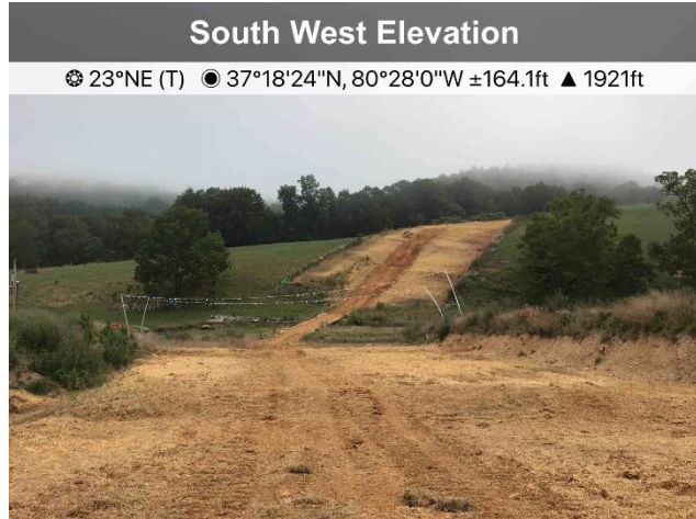
Fig. 1. St11354+00 areas has been seeded and mulched.
