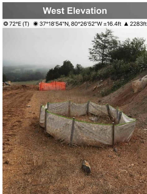
Fig. 3. Holes noted by Will Orndorff of DCR remain protected near MP 216.3
