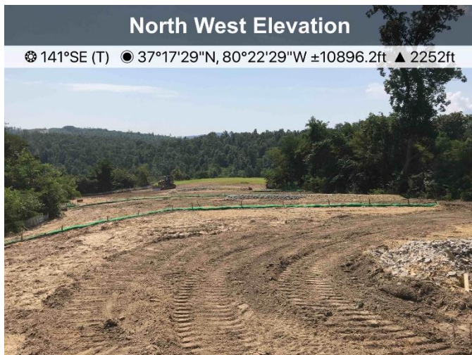
Fig. 3. Final stabilization efforts at St117838.
