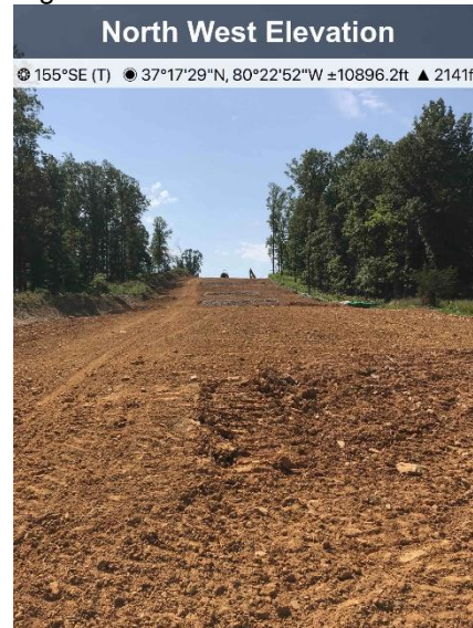
Fig. 2. Final stabilization efforts at St117818.
