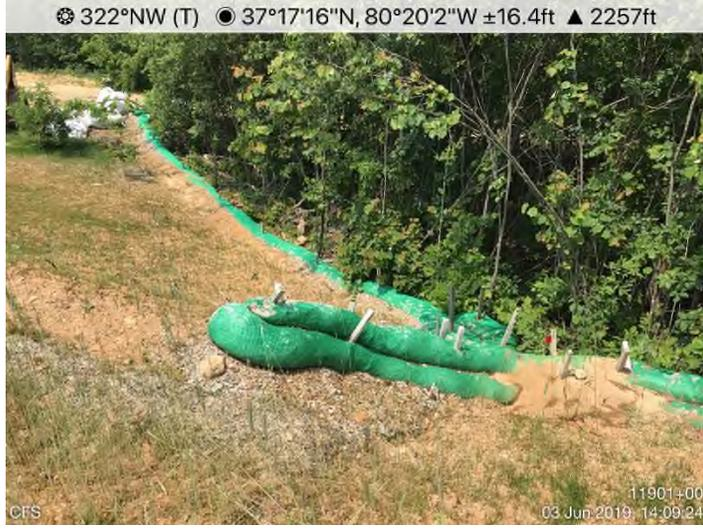
**Fig. 8: STA 11889+00 – Maintain/cleanout CFS.**
