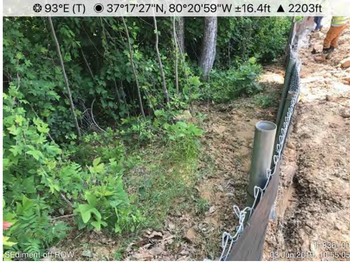
**Fig. 4: STA 11837+00 – Maintain/cleanout SSF.**
