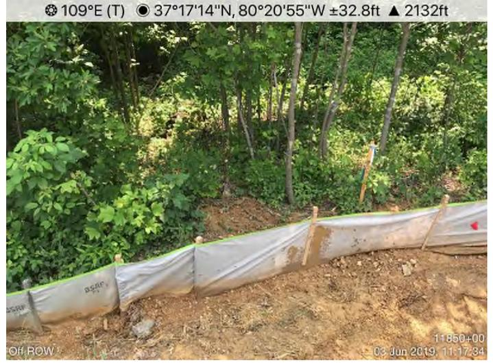
**Fig. 7: STA 11901+00 – Maintain/cleanout CFS.**
