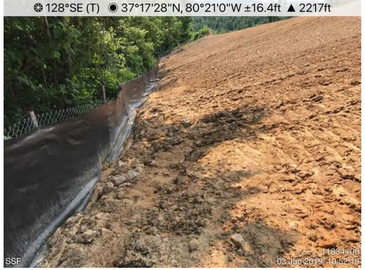
**Fig. 3: STA 11836+00 – Sediment off ROW.**
