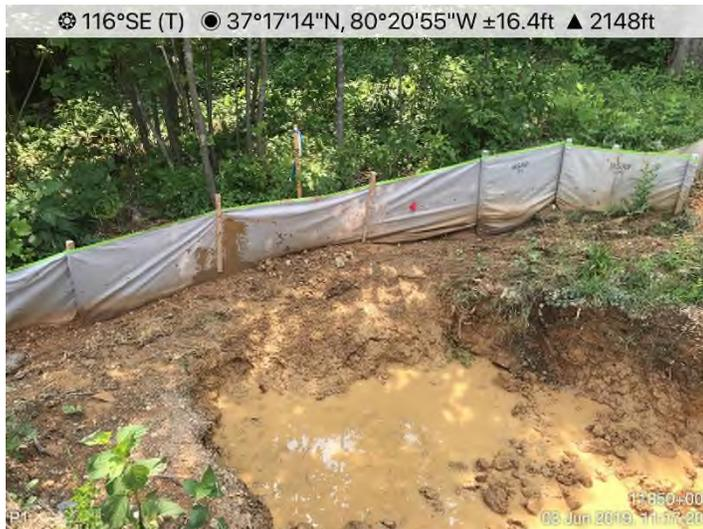
**Fig. 6: STA 11850+00 – Sediment off ROW.**
