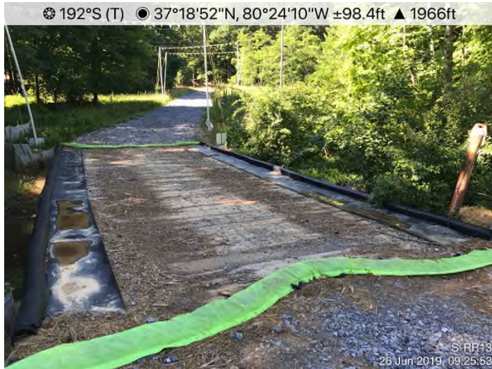
Fig. 3: STA 11165+00 – Controls in place. Area stabilized.
