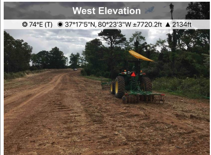
Fig. 4. Near MP 223 tractor for disking of soil on site
