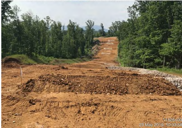
Fig. 3: STA 11826+00 – Controls in place. Permanent waterbar installation prior to subsoil disking.
