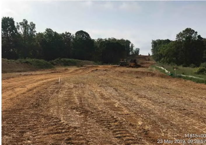
Fig. 3: STA 11826+00 – Controls in place. Permanent waterbar installation prior to subsoil disking.
