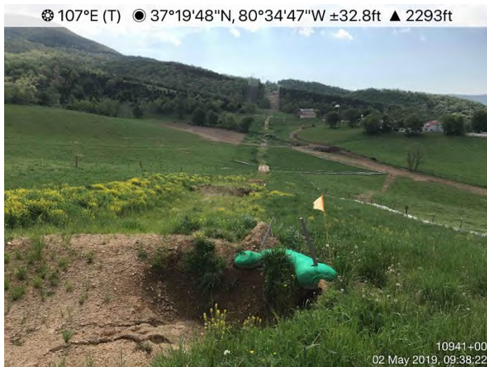
Fig. 3: STA 10985+50 – Stabilize erosion CIS stream S-E24.
