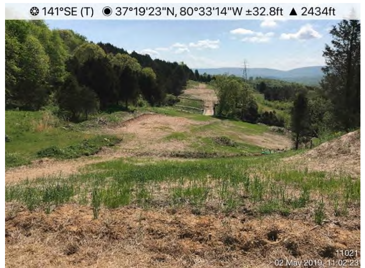
Fig. 4: STA 11021+00 – Controls in place. Area stabilized.
