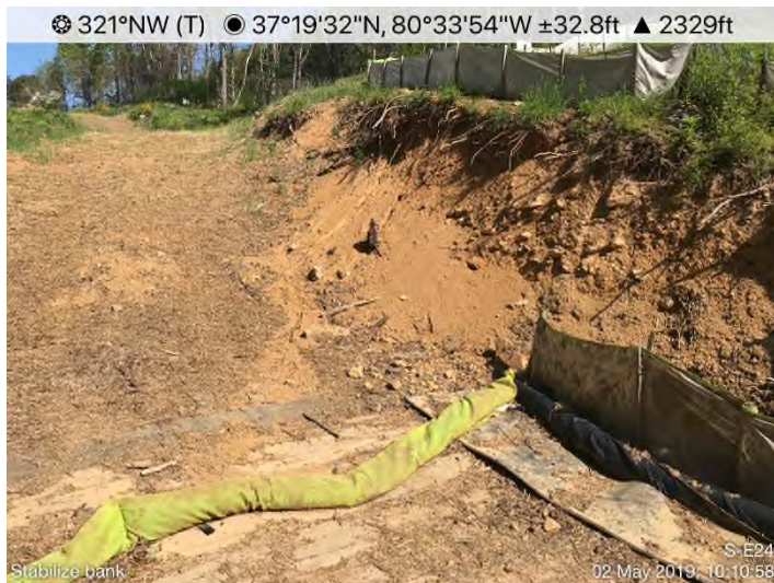
Fig. 3: STA 10985+50 – Stabilize erosion CIS stream S-E24.
