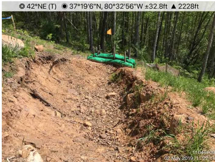
Fig. 7: STA 11120+00 – Waterbar maintenance needed.
