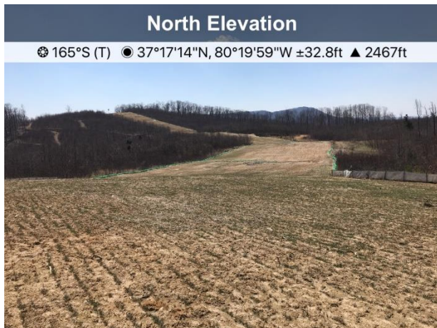
Fig. 3 St#11905+37 permanently graded area
