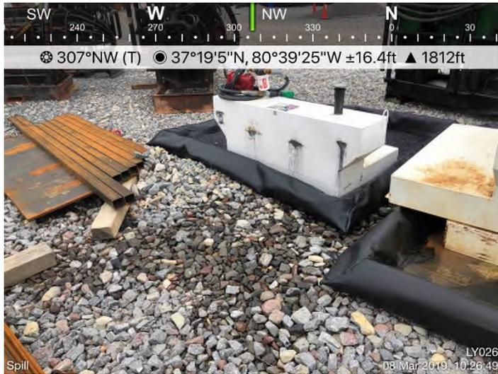
Fig. 2: LY 026 – Secondary containment maintenance needed.
