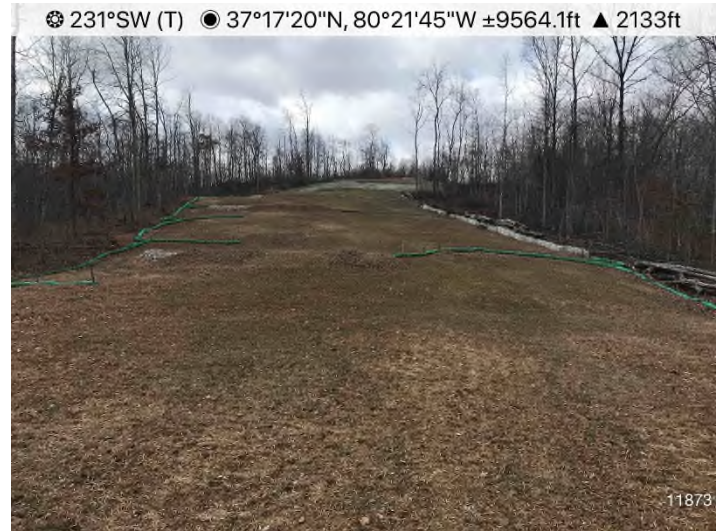
Figure 4: STA 11834+00 – Controls in place and functioning properly.
