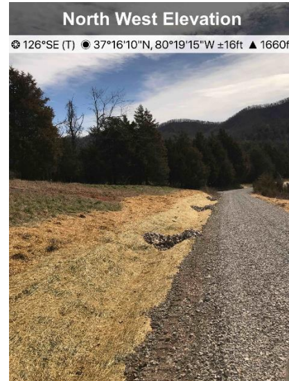
Figure 4: On AR MN-266, recent blanket matting and check dams have been installed in the ditch line.
