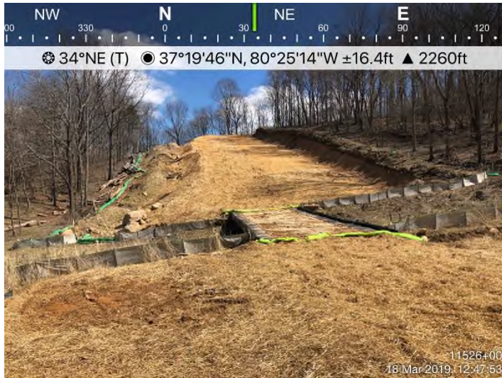
Fig. 7: STA 11507+00 – Area adequately stabilized. Controls in place.
