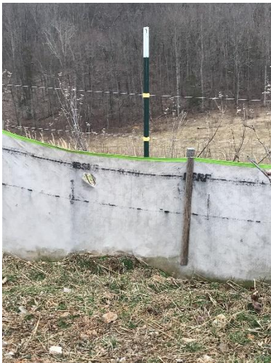
Fig. 3 St#11311+50 hole in P1 fence
