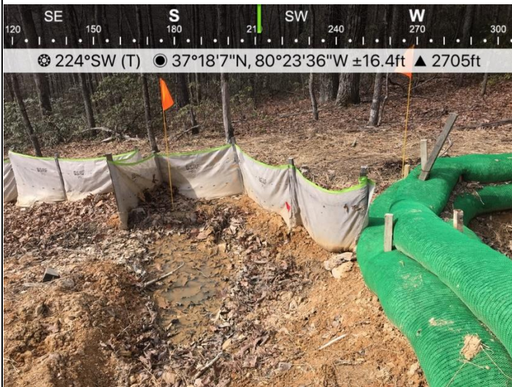
Fig. 3 St#11679+40 sump triple stack is undermined
