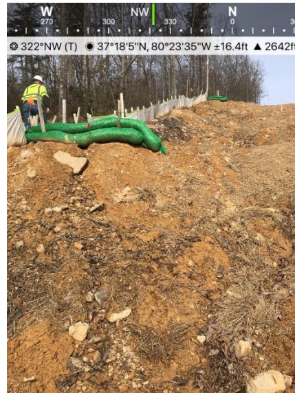
Fig. 4 St#11686+81 SS fence is undermined
