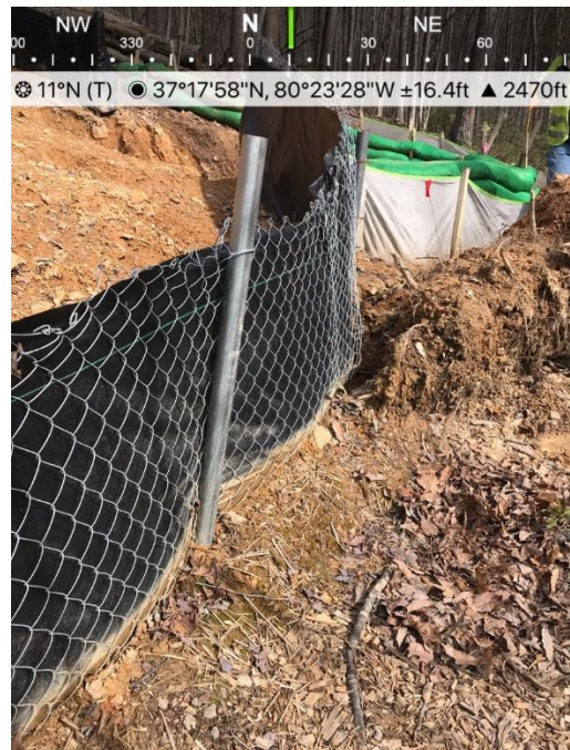
Fig. 4 St#11686+81 SS fence is undermined
