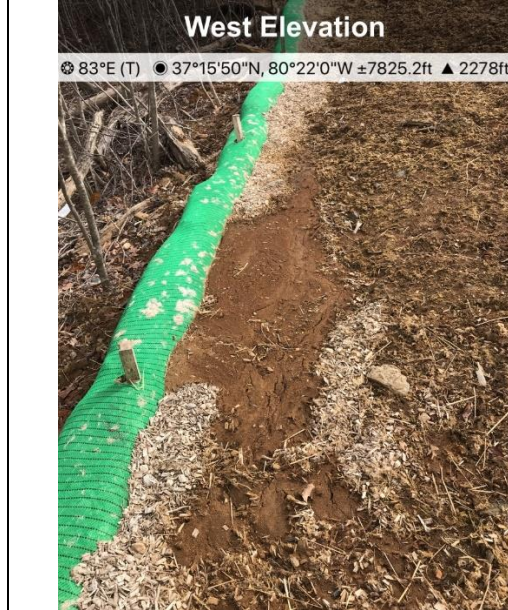
Fig. 4 Near St#11940+00 permanent waterbars have been installed
