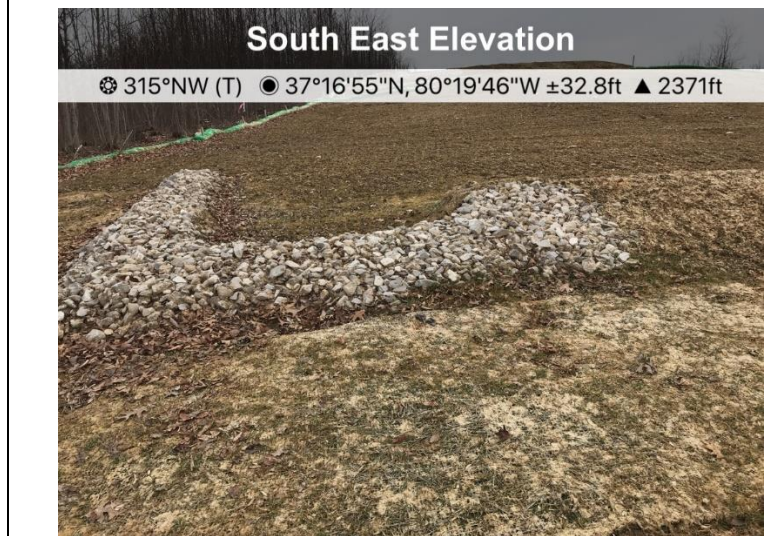
Fig. 4 Near St#11940+00 permanent waterbars have been installed
