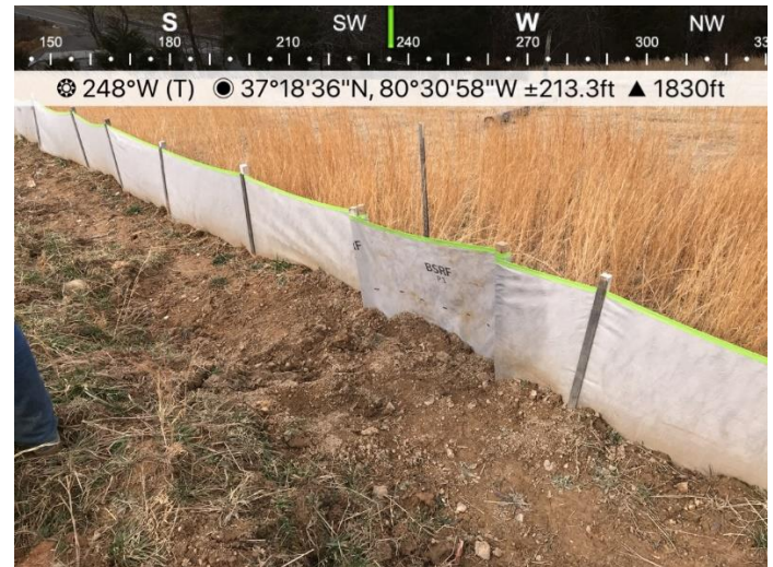
Fig. 4 At St#11172+48 P1 control has been repaired.
