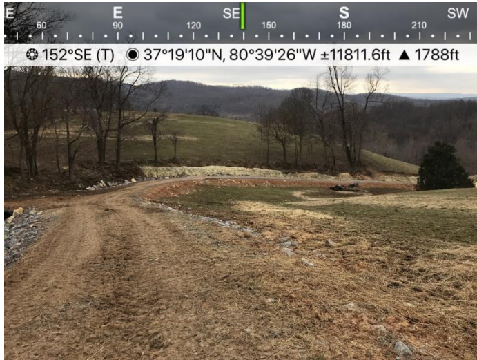
Fig. 1 Access Road GI-234, controls in place.
